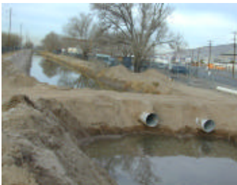
Picture 2: Ponding Site Two
