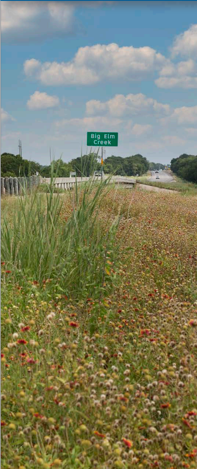
Big Elm Creek bridge at US 77. Photo by Lucas Gregory, TWRI.
