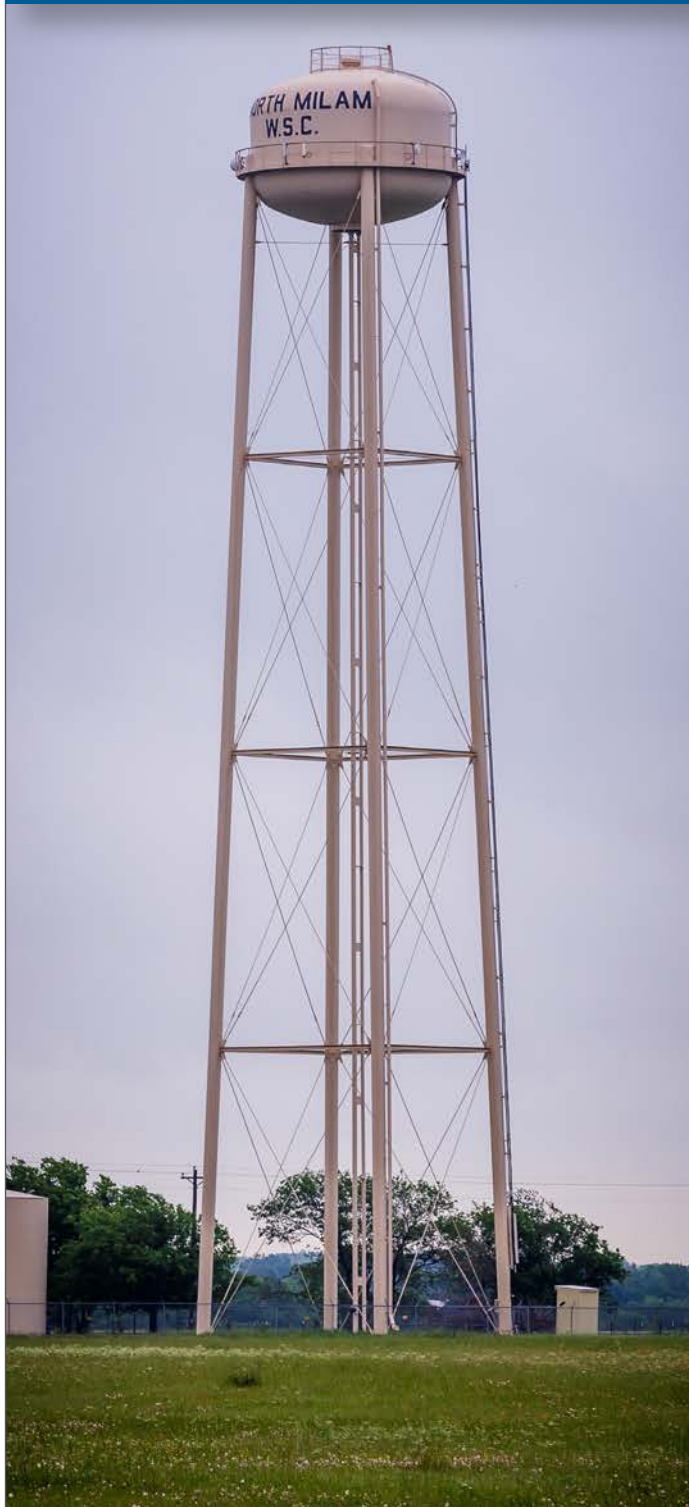
Rural water tower on FM 485. Photo By Ed Rhodes, TWRI.
