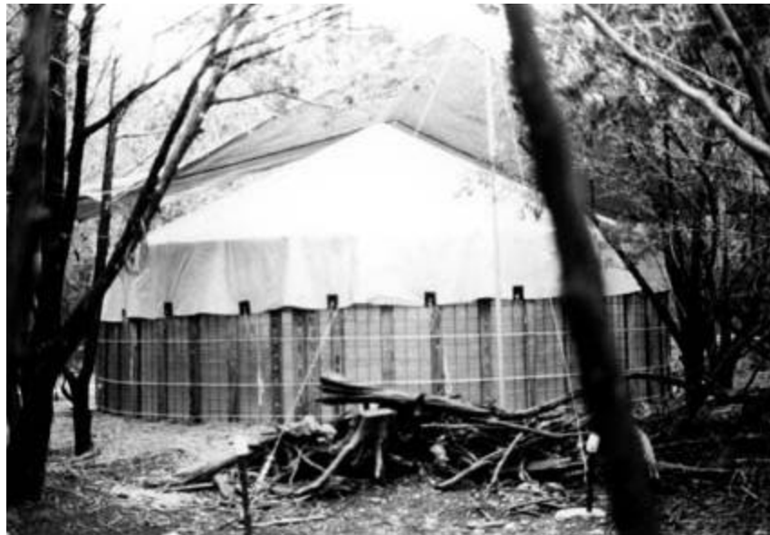
This 10,700-gallon tank was home-built by Mike McElveen from a stock panel form and sheet metal. Lined with polyethylene film, it stores rainwater for residential use.
