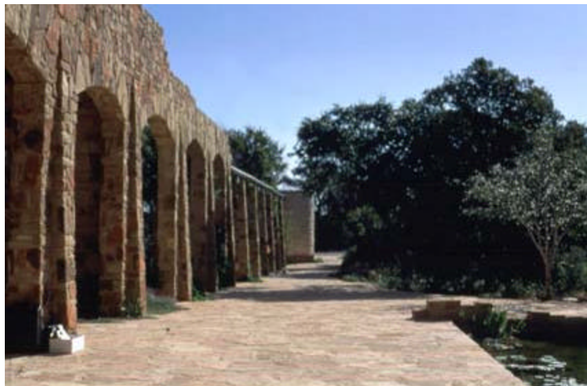
At the National Wildflower Research Center in Austin, a network of aqueducts conveys water from collection surfaces to cisterns. The 6,000-gallon Entry Cistern shown here is connected to a drip irrigation system.
