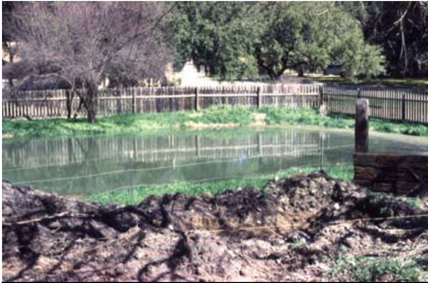
This one-half-acre, 8-foot-deep pond stores reclaimed water for irrigation of Fort Clark Spring's 18-hole golf course. It is located adjacent to a residential area.
