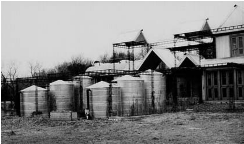
Galvanized steel tanks, integrated into the aesthetics of this demonstration home, provide 13,700 gallons of rainwater storage at the Center for Maximum Potential Building Systems.
