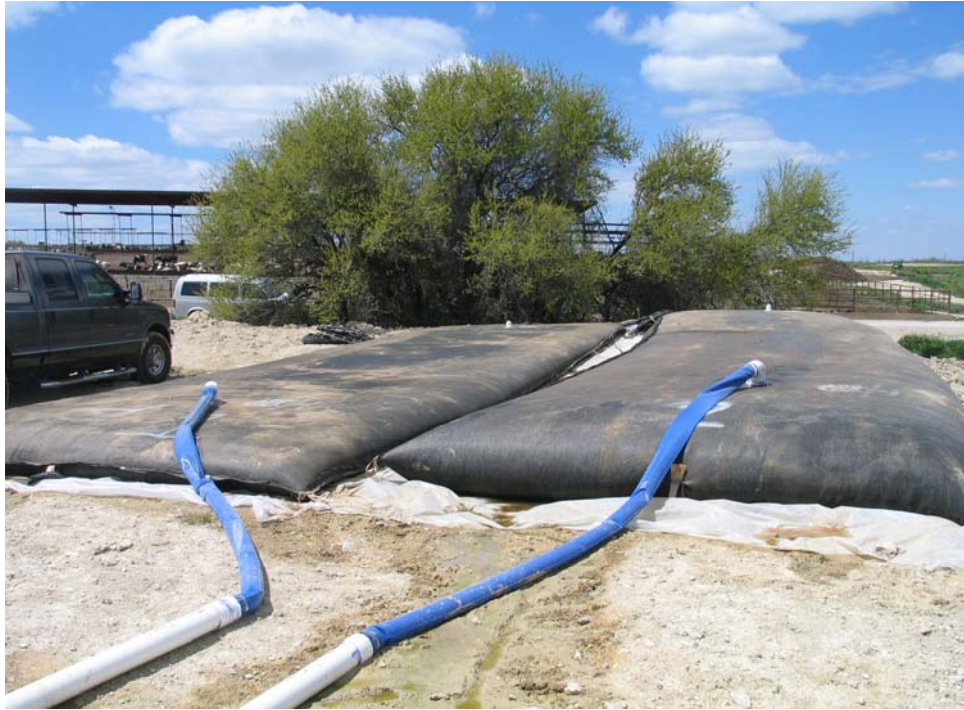
Figure 1. Partially filled Geotubes
