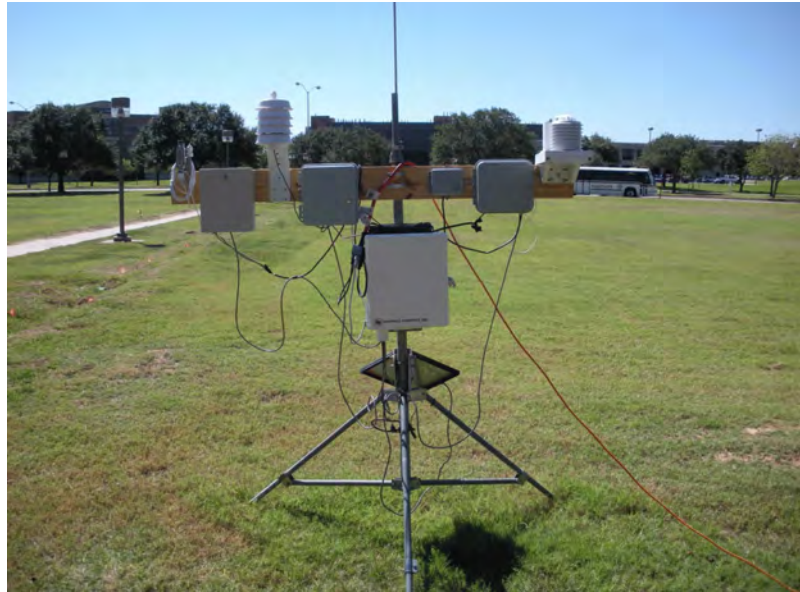
Figure A-4. Outdoor Tested Controllers
