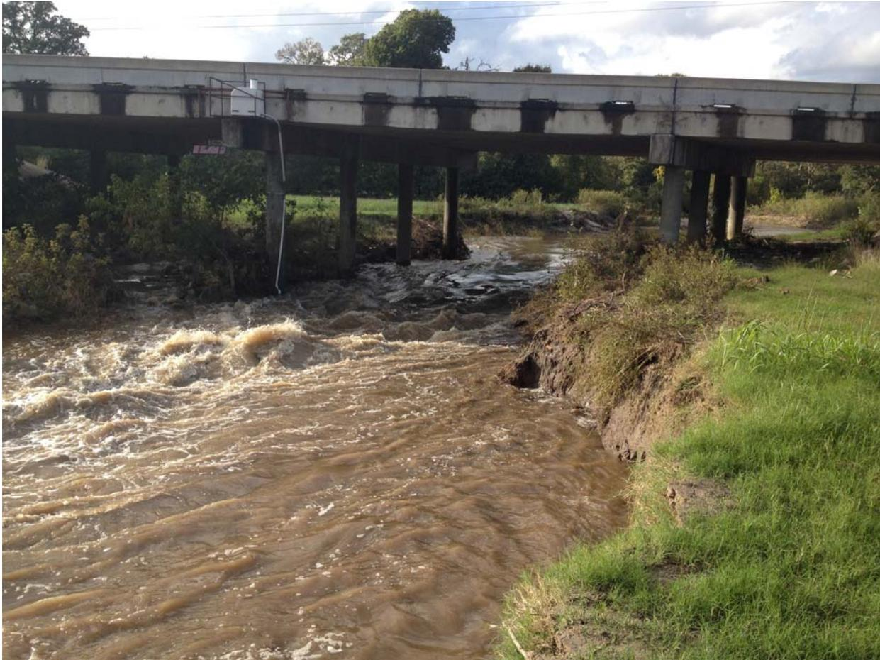
**High flow event on Carters Creek at WM D. Fitch Pkwy (Station 21259) in October 2013. Events such as this have caused severe erosion at this site as is evidenced by the near vertical creek bank on the right side of the photo.**
