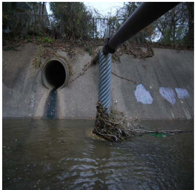
Storm Drain Outlet and Adjacent Wastewater Line
