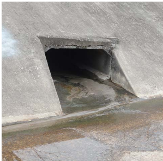
Sediment in Storm Drain Outlet
