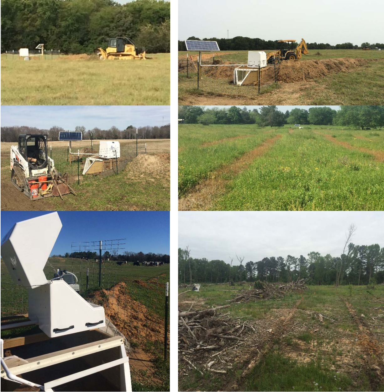
Figure 3. (clockwise from top left): Texas A&M Forest Service constructing earthen berm; completed earthen berm around farm-scale site; field scale plot with silvopasture and grazing management practices applied; field scale forest stand establishment plot (seedlings planted in furrows); farm scale control site (continuous grazing ~40 AUs); completed berm repairs following large rain event
