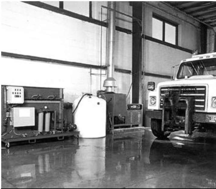
This water reclamation system is installed for the Brazos Transit System. The system will kill bacteria. Water and soap are separated and reused.
