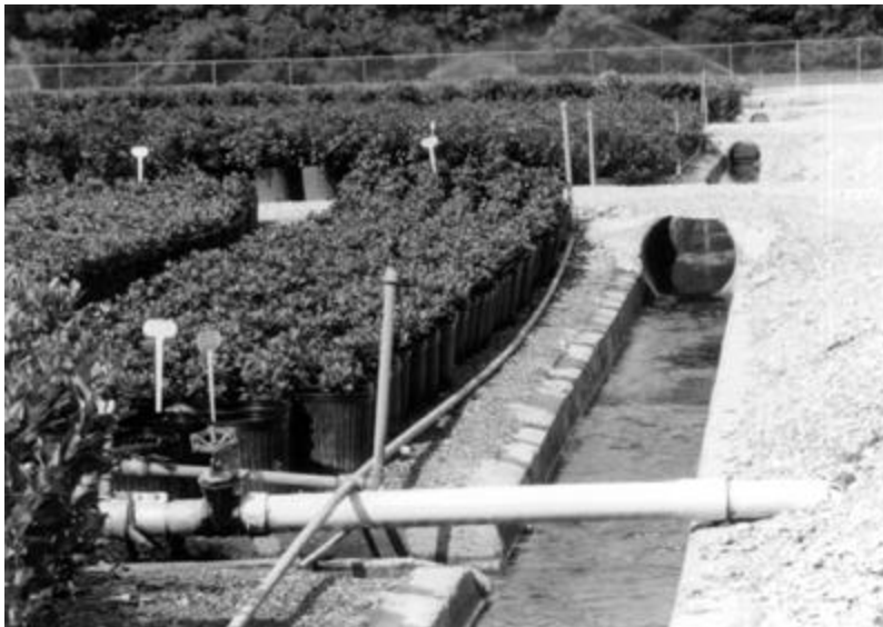
A series of concrete and plastic-lined ditches carry excess runoff to a central treatment area where the water is cleansed of organic matter, suspended solids and bacteria.
