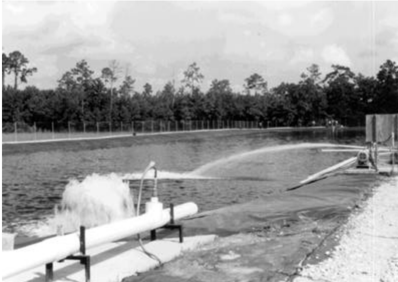
A large holding pond stores reclaimed runoff water and ground water for irrigation of nursery plants and trees. the tank is lined with high-density polyethylene to reduce percolation loss.
