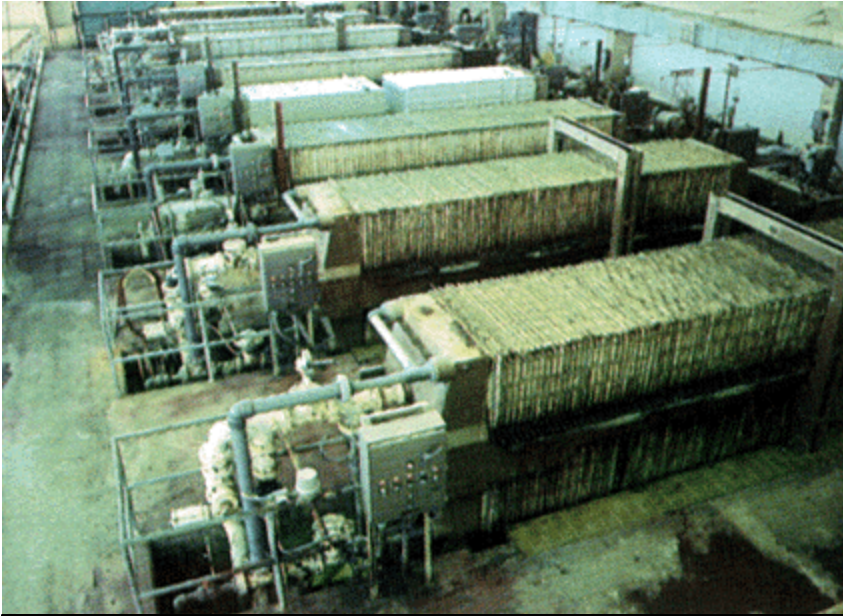
Sludges are blended with lime, chemically stabilized, and thickened in large filter presses to a dryness of about 34 percent in the sludge dewatering process.
