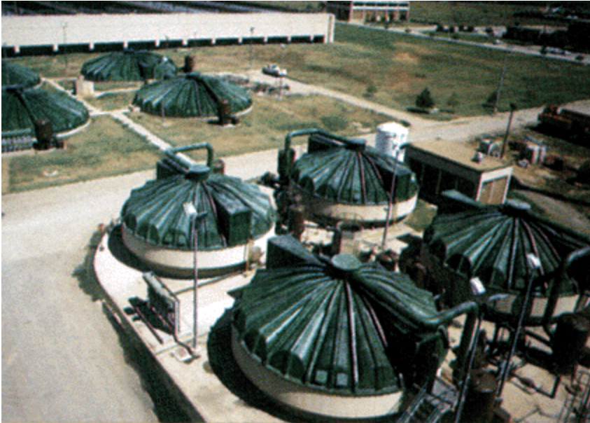
Primary sludge (solids separated by gravity) and secondary sludge produced by the activated sludge process are thickened in gravity and dissolved air floatation thickeners.
