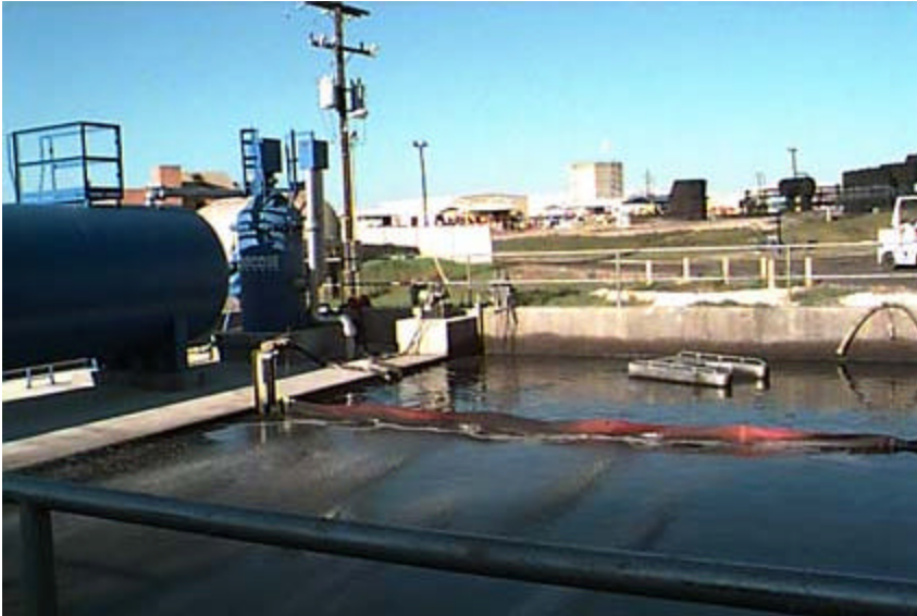
In the oil-water separator, the mixture passes through a bar screen, pan skimmer, pre-coalescer (which coagulates emulsified oil), and finally the oil/water separating unit.
