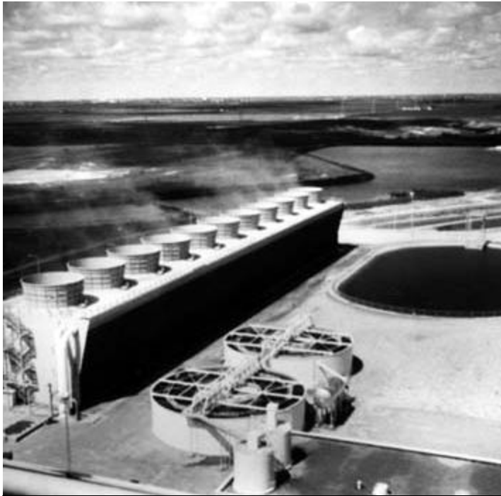
The 486-megawatt, natural gas-fueled Jones Station in Lubbock has used treated wastewater in its cooling towers since 1971. Southwestern Public Service estimates use of secondary treated wastewater conserved almost 75 billion gallons of water in 1980.
