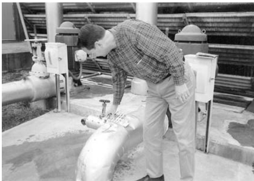
Security DBS Maintenance Supervisor Les McDarty checks a valve at one of the plant's cooling towers.
