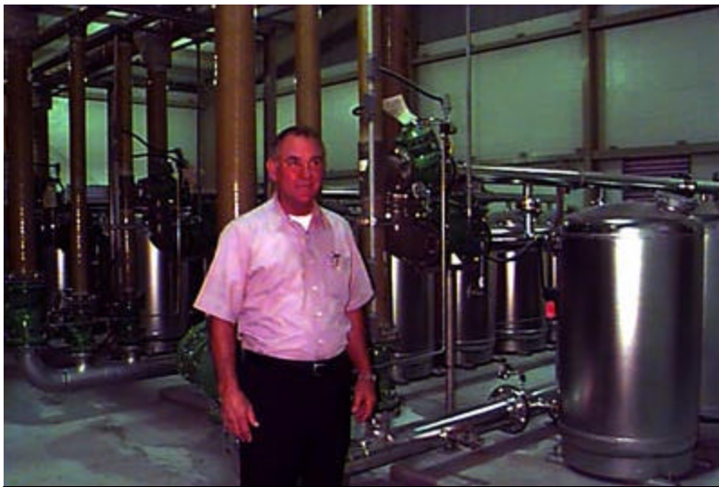
Harlingen Water Works System Engineer Dennis Raymond in the pressurized sand filter plant installed by Harlingen Water Works to filter wastewater in preparation for reverse osmosis and eventual delivery to the adjacent Fruit of the Loom factory. This 66-tank installation is the largest in existence.
