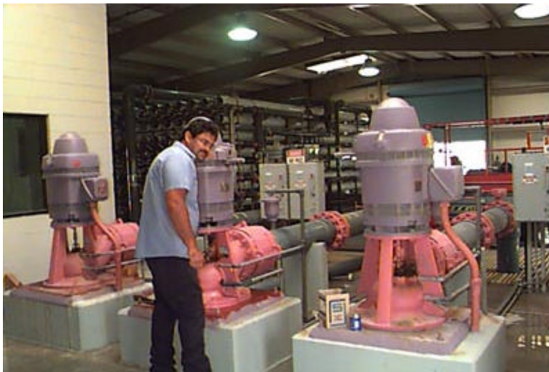
Harlingen Water Works Technician Javier Trevino prepares to work on purple pumps which move reverse osmosis (RO) treated wastewater to storage tanks. RO membranes are seen in the background. The RO plant has a present capacity of 2 mgd, which will soon be doubled.
