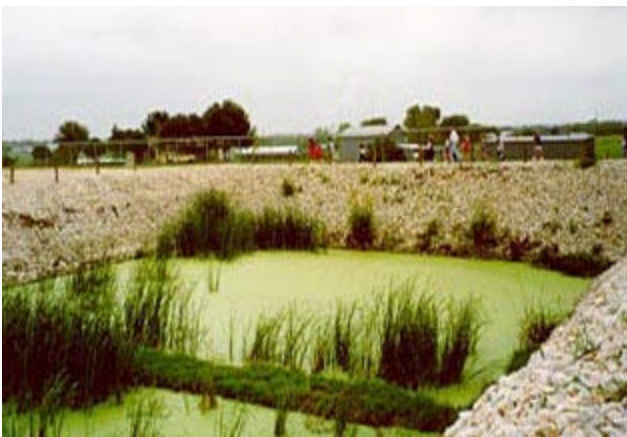
Part of the habitat created by the constructed wetlands at Heritage Middle School is the marsh.
