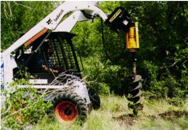
Certified on-site septic facility installer Randy Bendele, owner of Benke Septic Systems, Inc. bores a test hole with an auger as part of the permit process for a new residential OSSF on the outskirts of San Antonio.
