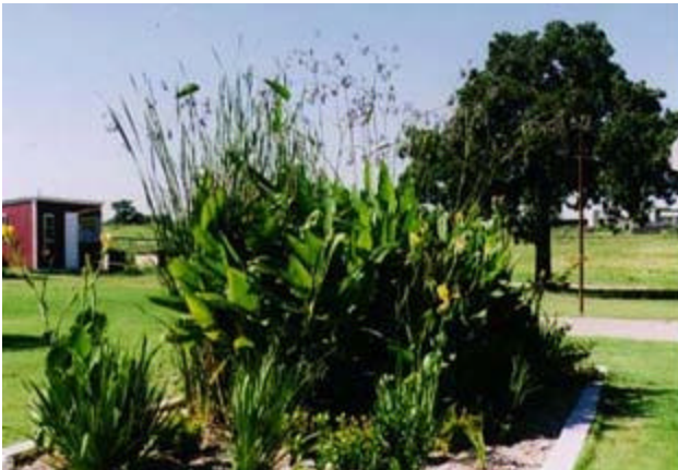
Canna lillies planted in a gravel medium form a filter for wastewater in this constructed wetland on-site septic facility.
