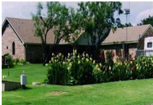
The constructed wetland on-site septic facility can be incorporated as an attractive landscaping element, as at this house in Temple.
