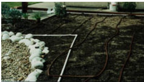
Driplines are installed prior to planting of vegetation at the Johnson Space Center.
