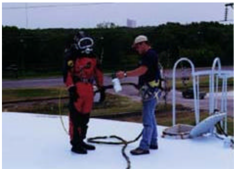
Diver Mike Erinakes of U.S. Underwater Services Inc. is sprayed with a disinfectant solution before entering a water tank on the Texas A&M University campus in College Station.
