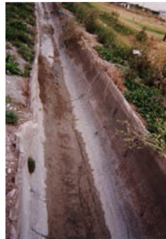
Improvements to canals such as this one in the Lower Rio Grande Valley will mean a net increase in available water due to lessened conveyance losses.
