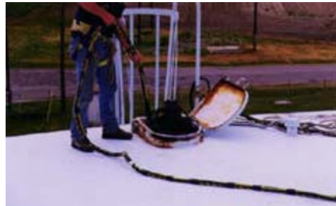
Down the hatch! The technician feeds the tether as the diver descends into the tank. The tether contains a light cord, video cable, and audio cable, which allow for communication between the diver, the technician with the tether, and the technicians in the truck.
