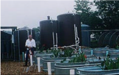
Texas A&M University horticulturist Garry McDonald poses amid constructed wetland cells which cleanse irrigation runoff prior to reuse. In the background are two 2,000-gallon storage tanks.
