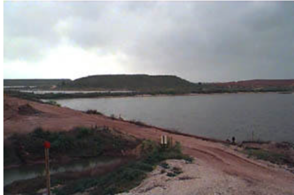
At the Reynolds Alumina Plant, large impoundments capture rainwater for use in processing alumina from bauxite. The refining process does not require high-quality water, but cannot use saline water.
