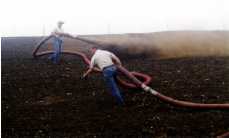
A.J. Wallace and Walter Struckman of Eco Mulch drag horses and spray manure-based compost on a steep highway right-of-way.
