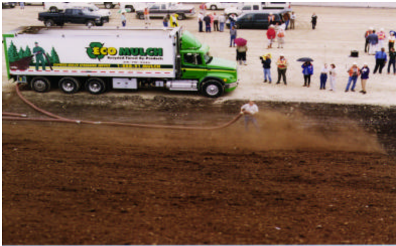
Compost is sprayed on a steep highway right-of-way on Texas 195 south of Killeen at a demonstration attended by state officials, dairymen, and commercial dirt and loam operators
