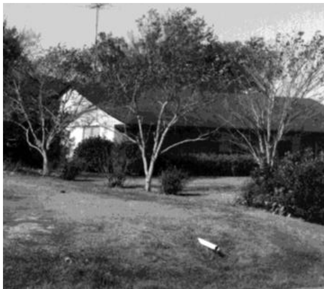
Part of this project involves identifying obvious areas where septic tank effluents are not being properly discharged. For example, this home (above) discharges septic wastes through an exposed pipe which may lead to runoff pollution.
