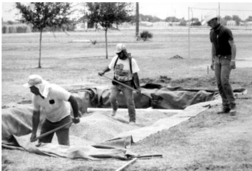
Workers place gravel in the bed of this rock plant filter at the Texas A&M Center at Weslaco.
