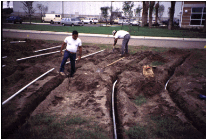
Workers in Westaco install lateral lines. The trenches are curved so that each lateral line is at a constant elevation.
