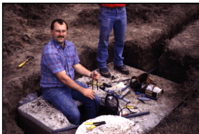
Bruce Lesikar (above) installs a pump that will provide a source of wastewater for supply and lateral lines.
