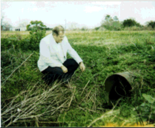
The LCRA looked for obvious signs that on-site wastewater systems were malfunctioning. Here, Ed Schulze of the Matagorda County Health Department examines raw or partially treated sewage that flows onto the surface.
