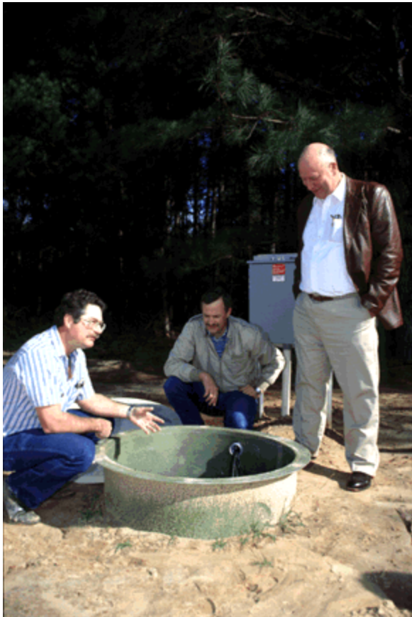
Stephan Gelwicks (far left), Ken Awtrey(middle), and John Herndon (far right) discuss how wastewaters will flow from the septic tank and sump into holding ponds
