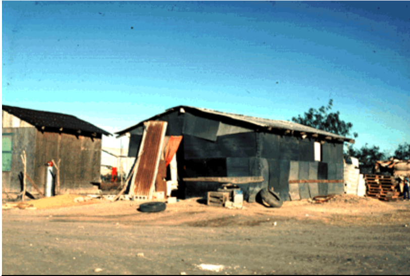
Many colonias include homes that lack even the most basic infrastructure and maintenance like this one. Only a few homes in colonias have adequate drinking water or on-site wastewater treatment.
