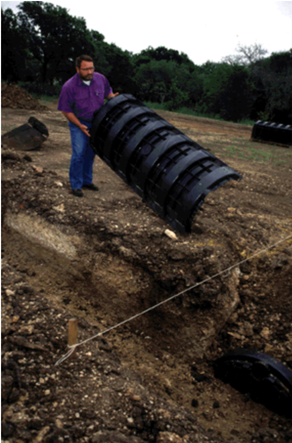
Dave Jensen helps install an infiltrator near the Eagle Mountain Lake Volunteer Fire Department. These systems feature a series of interlocking plastic panels and form a leaching chamber. They provide effective treatment but require a much smaller drainfield than conventional systems.
