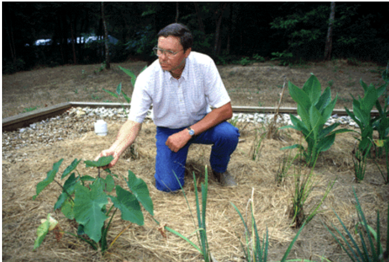
Melvin Adams of USDA/NRCS checks the progress of these wetlands plants that will help treat wastewater in this constructed wetland cell. A straw mulch has been spread to help lower temperatures and plant stress.
