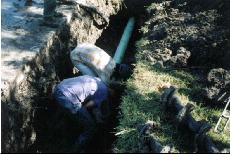
Workers install this small diameter sewer in Point Royal Estates. The sewer replaced conventional systems that were failing.
