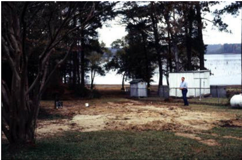
Doug Dowler of ANRA stands beside this on-site wastewater system near Lake Sam Rayburn.
