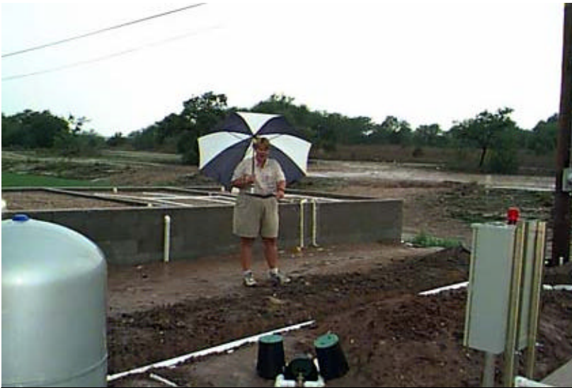
Sarah Calvert of the Austin Travis County Health Department inspects this innovative system.
