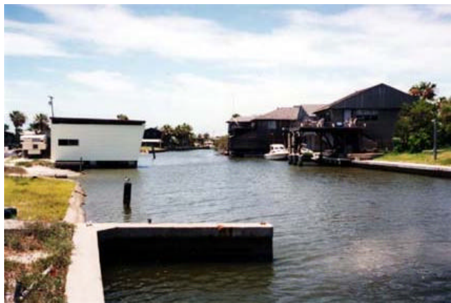
This photo shows on-site systems that were installed on small lots near the Texas coast.
