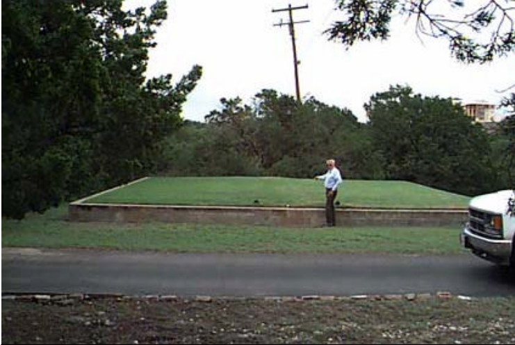
This photo shows an evapotranspiration bed, which for many years was a recommended strategy for on-site wastewater treatment. These beds are not used often anymore, though, because of high costs and performance problems.
