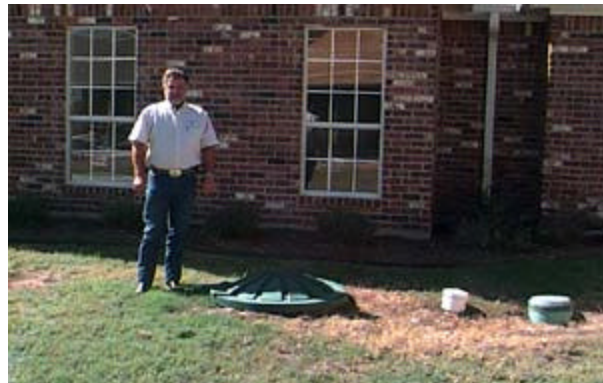
Dennis Musick, an inspector with Waco Water Utilities, stands beside this aerobic system which was installed at a new home. Many aerobic units are being installed along the Highway 84 corridor because problem soils often limit the use of conventional septic tanks and drainfields.
