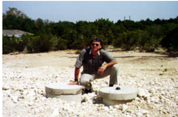
Paulo Pinto of the Williamson County and Cities and Health District oversees the installation of many non-standard onsite wastewater treatment systems like this one.
