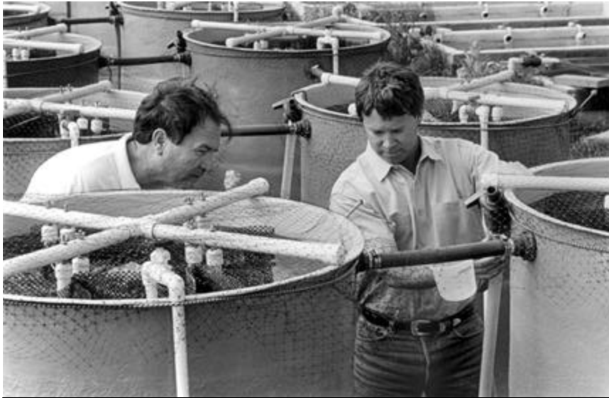
TCU biologists Durward Smith (left) and Ray Drenner monitor the performance of algae-eating fish in an innovative wastewater treatment system.
