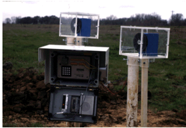
This control box is where groundwater data will be recorded so it can be downloaded.
