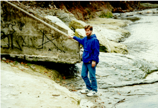
David Robertson stands next to a stormwater pipe which has been undercut by White Rock Creek. Urbanization of North Dallas has resulted in increased intensity of stormwater runoff events in the creek. The erosion of the channel sidewalls enhanced by the vigorous runoff events provides an unlimited supply of sediment which is filling up White Rock Lake.
