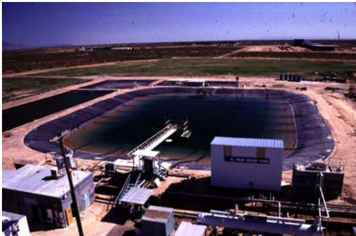
This photo displays a saline solar pond at the University of Texas at El Paso developed by John Walton and Andrew Swift. The pond produces energy from salt water.
