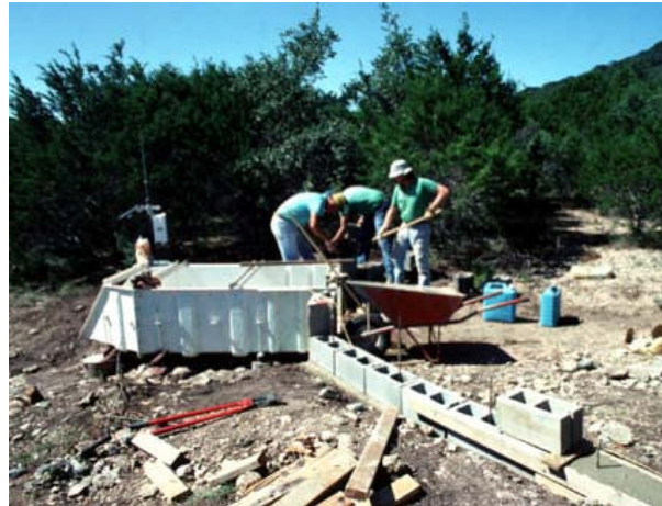
Researchers with the Texas Agricultural Experiment Station's Blackland Research Center at Temple install this flume to measure runoff from plots where nuisance brush species were removed.
