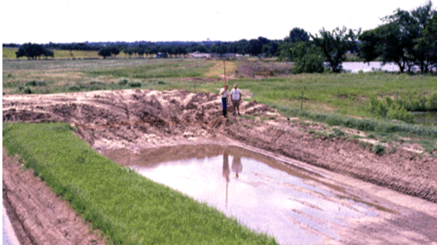
A newly dug wetlands cell at TAES Stephenville. This cell will be planted with wetlands species to treat agricultural wastes.
