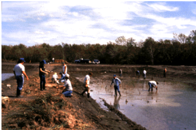
Workers with the Tarrant County WCID plant this wetland, which is designed to improve water quality.
