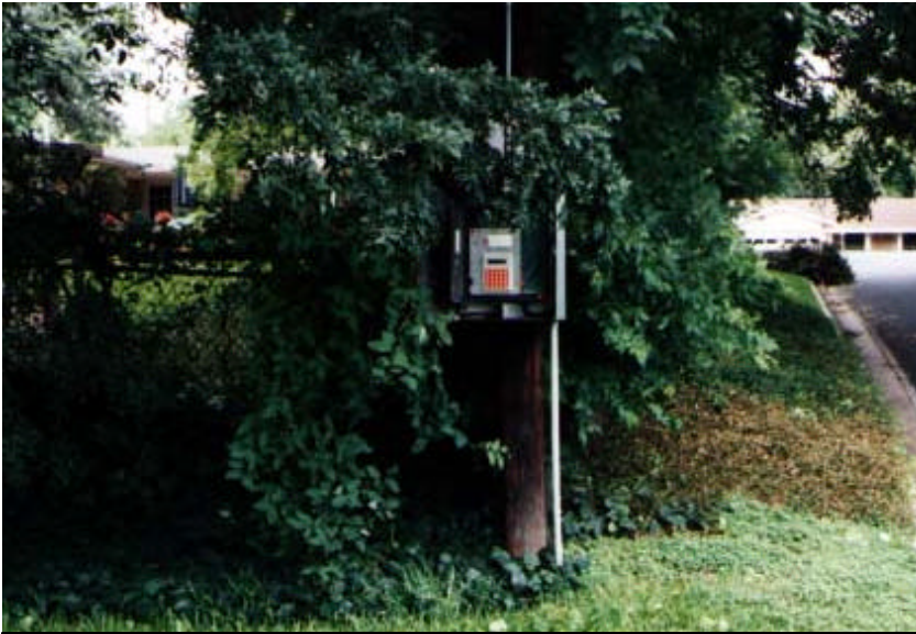
The City of Austin used devices like this one to transmit data on hourly water flows to a central computer. The system provided insights on water use in different neighborhoods that was essential for planning and rate setting.
