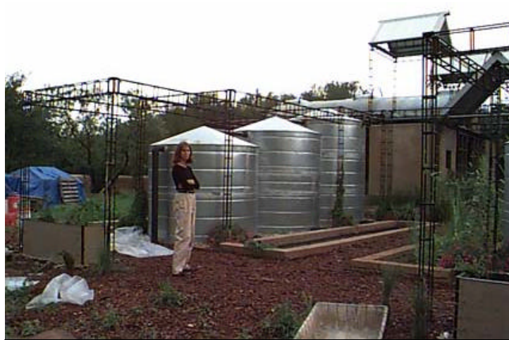
Gail Vittori, who wrote the handbook, stands near some cisterns used as part of a prototype rainwater harvesting system at the Center's site east of Austin.
