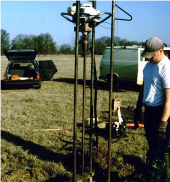
This photo shows the installation of the hydrology field lab at Texas A&M University - Commerce.
