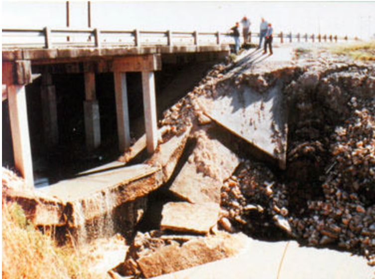
TTI researchers have developed a better method to predict scour that may lessen damages at bridges like this site in East Texas.
