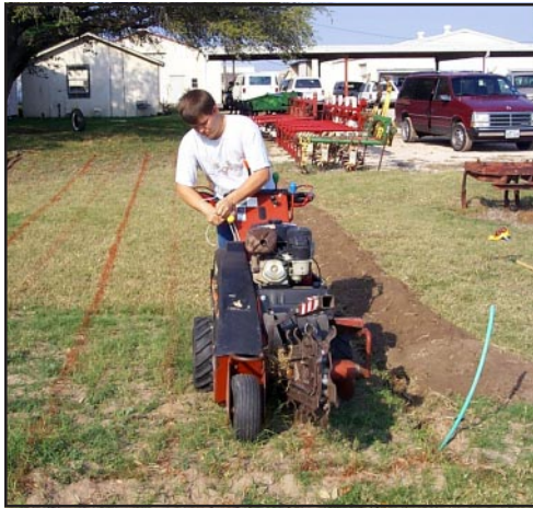
Photo by Vance Weynand, TAMU Vance Weynand installs this drip irrigation system.
