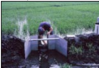
Water is often distributed to rice fields through canals and gates like this one.
