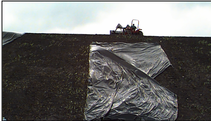
TTI staff members install an erosion control blanket on this man-made hill at the TAMU - Riverside campus this spring. TTI uses the site to test how well various materials retard erosion.
