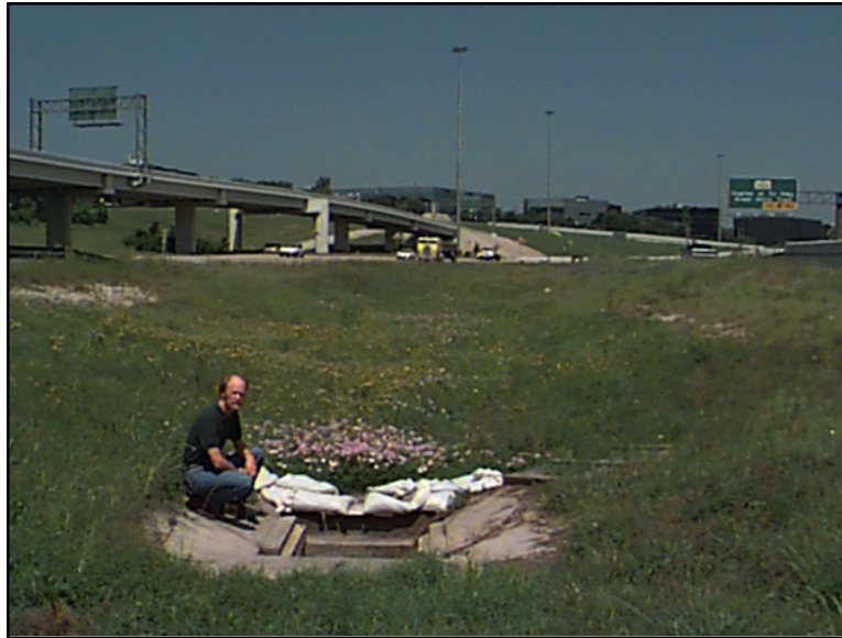
Mike Barrett of UT Austin shows how this vegetated area can trap runoff pollutants and sediments. This site is on the MoPac Expressway in Austin.
