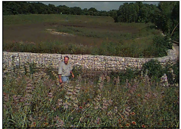
Roger Glick of the City of Austin stands in front of this rock berm that diverts stormwater runoff into a wet detention basin.
