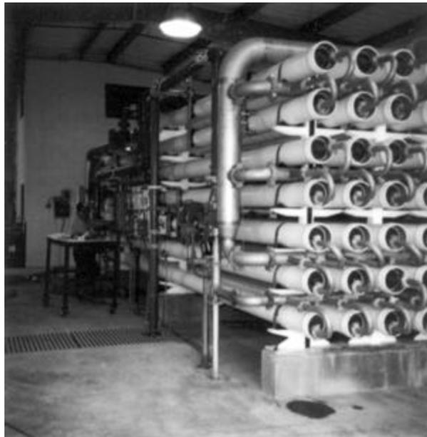
*This pressurized flow-through filter system is part of the Reverse Osmosis treatment facility at the City of Harlingen Water Works. RO-treated water is reused by Harlingen's Fruit-of-the-Loom plant in its partnership with the City of Harlingen.*
