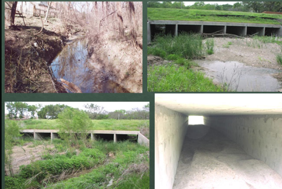
Poorly designed road crossings / bridges
