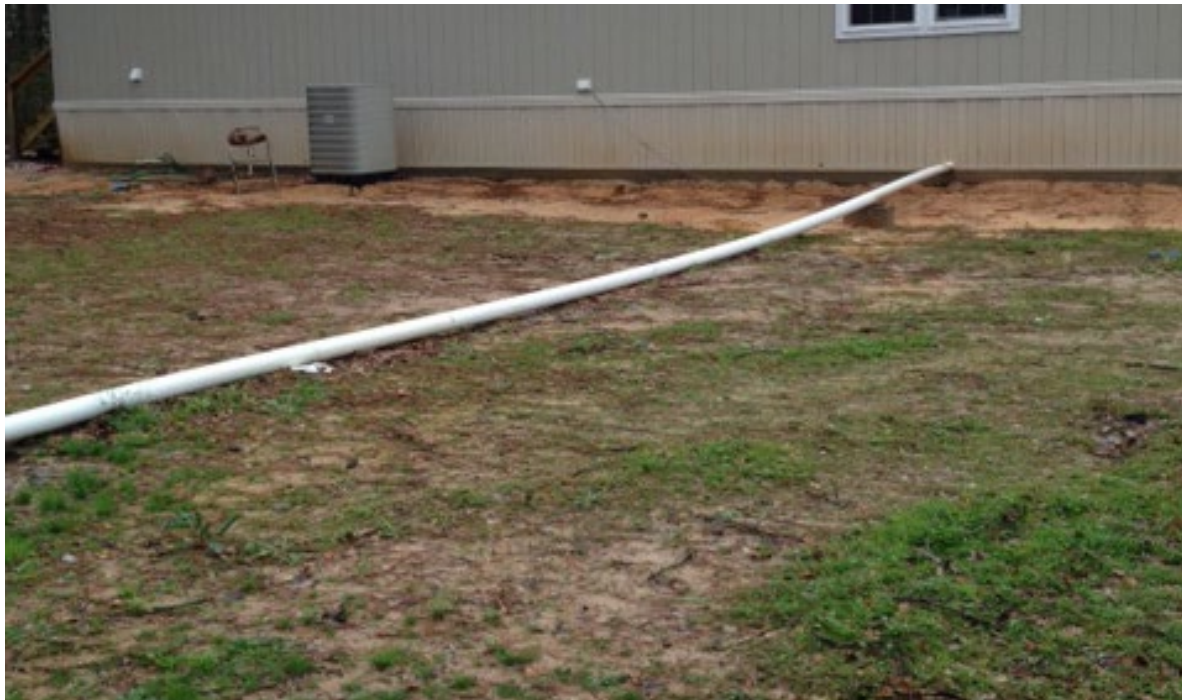
Below: Drainpipe coming from toilet inside residence.
