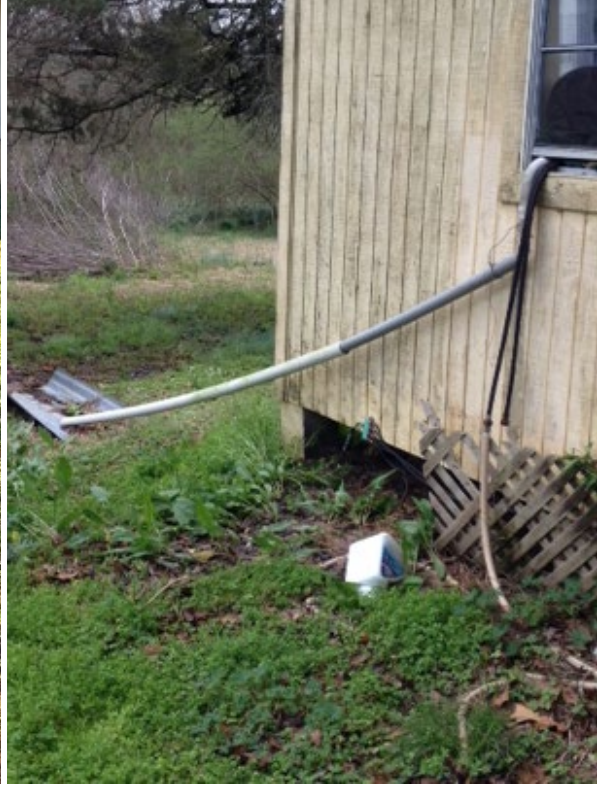
Above, left: Drainpipe coming from toilet inside residence. Standing sewage water near house.
