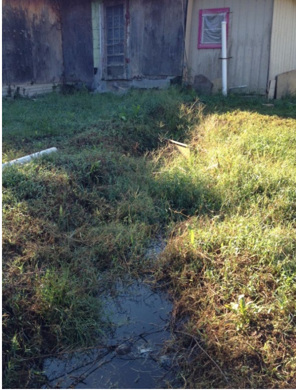
Above, left: Drainpipe coming from toilet inside residence. Standing sewage water near house.
