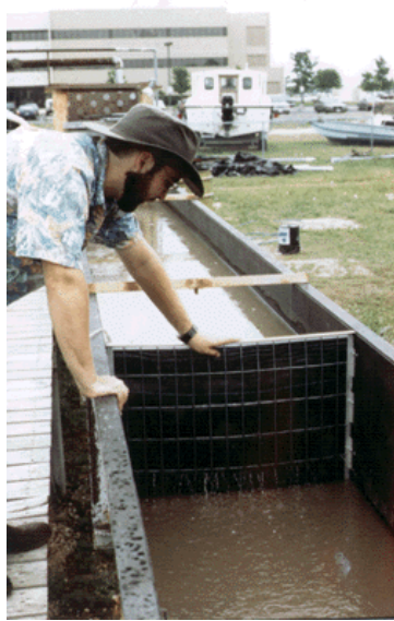
UT student Ty Lehman checks the performance of this geotextile fence that is designed to trap sediments.
