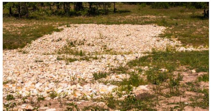
The stabilization of areas frequently and intensively used by people, animals, or vehicles by establishing vegetation cover, surfacing with suitable materials, and/or installing needed structures
