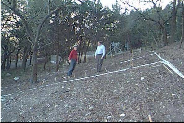
*George Witta of Wittaworks Construction of Elgin installs this aerobic drip emitter system that Sherman Hart designed. The system is on a steep slope in West Austin and utilizes drip irrigation to efficiently dispose of effluents.*
