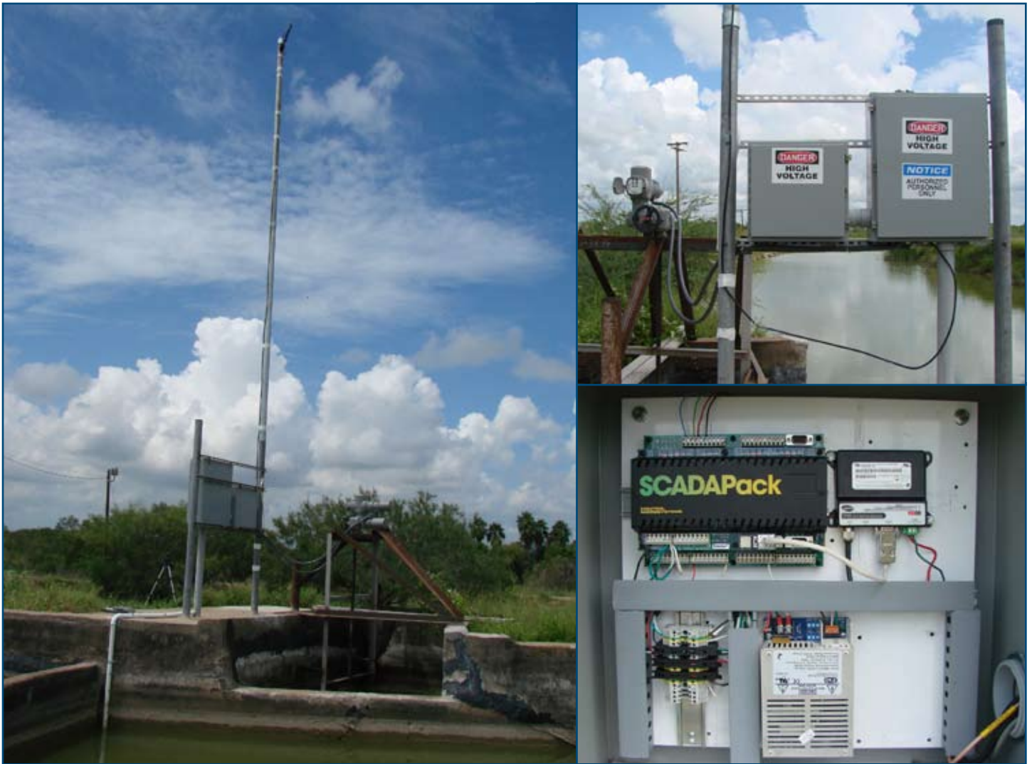
Left: Emergency Gate and Remote Terminal Unit (RTU) site. Right: The components of the Remote Terminal Unit.
