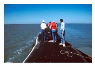
ultraviolet light, which otherwise would deteriorate them. The intent is that these larger geotubes would protect open embayments from the erosive effects of waves. In addition, smaller, polyester, geotubes with diameters of 7- and 15-feet are being deployed to protect earthen marsh terraces from slumping and erosion. Both types of geotubes are anchored by tons of material dredged from the bay. The half-life of both types of geotubes is expected to be roughly 20 years.
