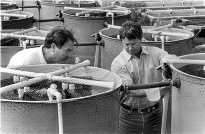
TCU biologists Durward Smith (left) and Ray Drenner monitor the performance of algae-eating fish in an innovative wastewater treatment system.
