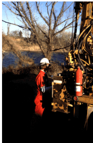
Part of the project involves using a device that sends heat impulses into the ground so that 3-dimensional groundwater flow patterns can be traced.
