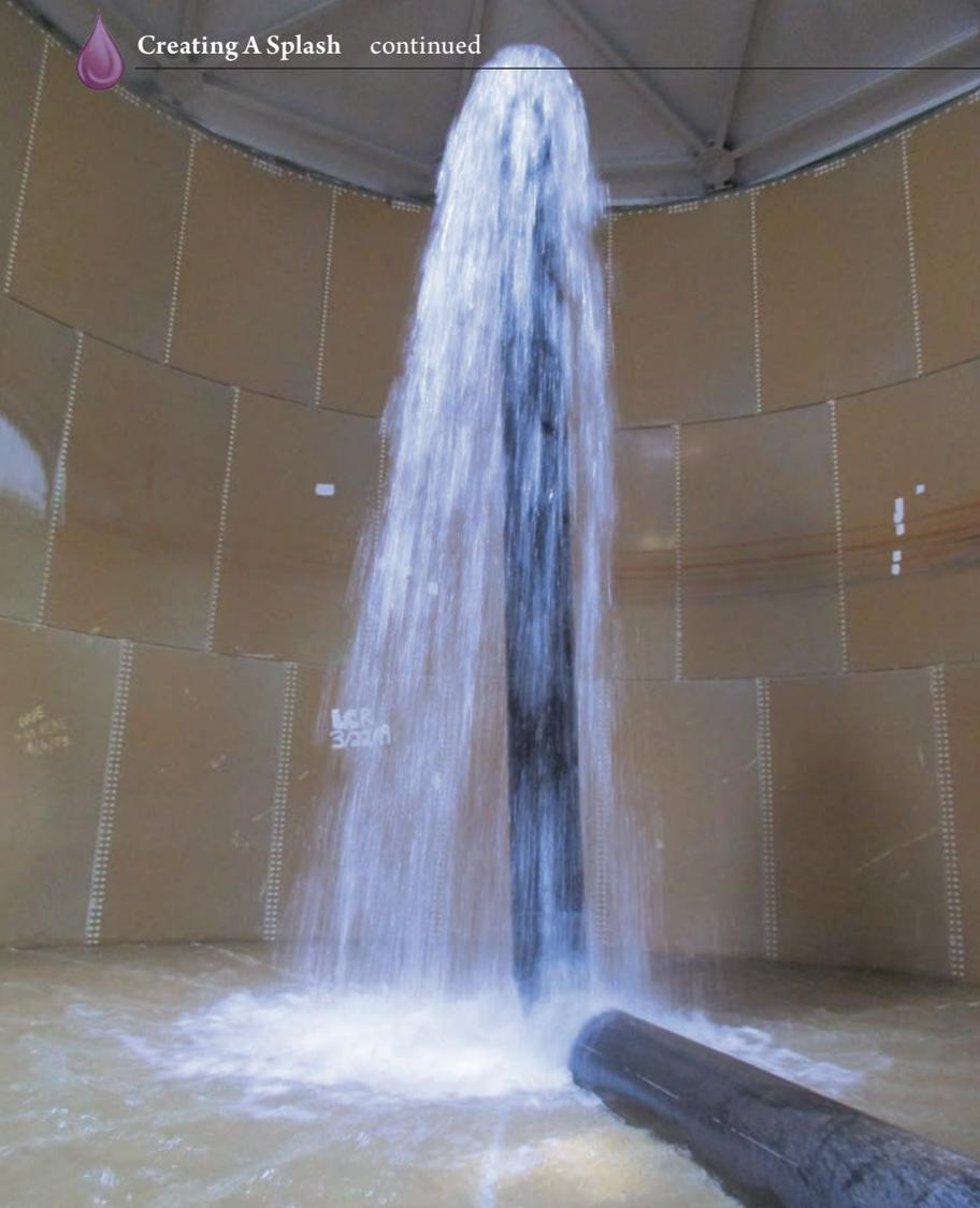
The city created a splash pump with spray heads. When water from the spray heads splashes down on the water in the tank, the impact dissipates the total trihalomethanes. Photo courtesy of the city of Lago Vista.
